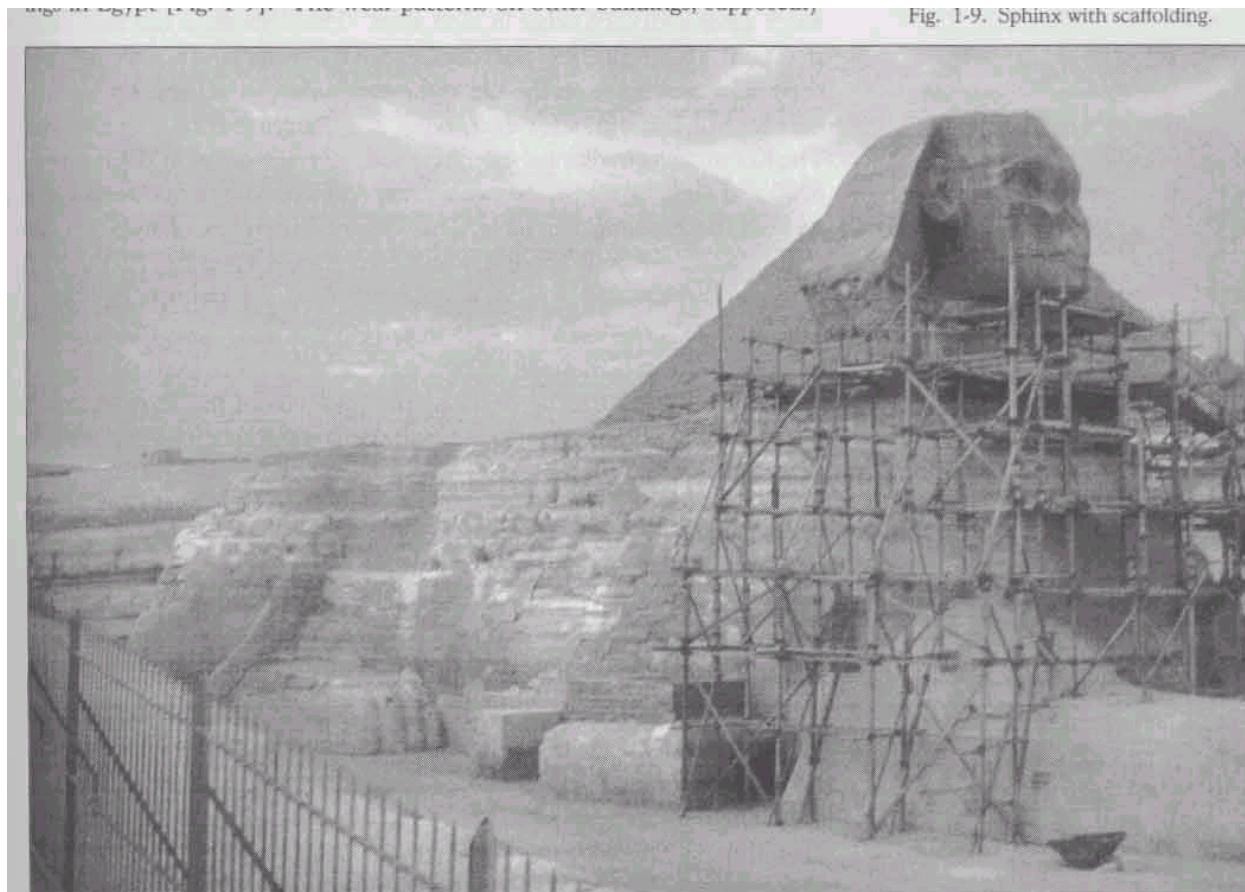
Fig. 1-9. Sphinx with scaffolding.
